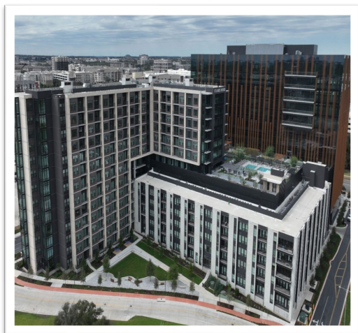
Uptown ATX - Block A Construction | 652,404 SF | Austin, TX
